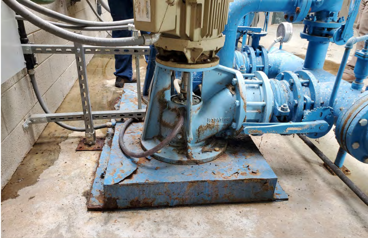
Figure 3-19: Return Pump Skid
