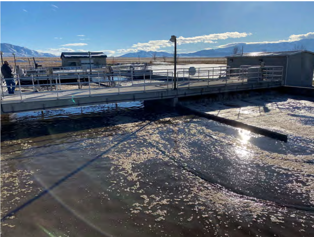
Figure 3-6: Oxidation Ditch Foaming – High MLSS
