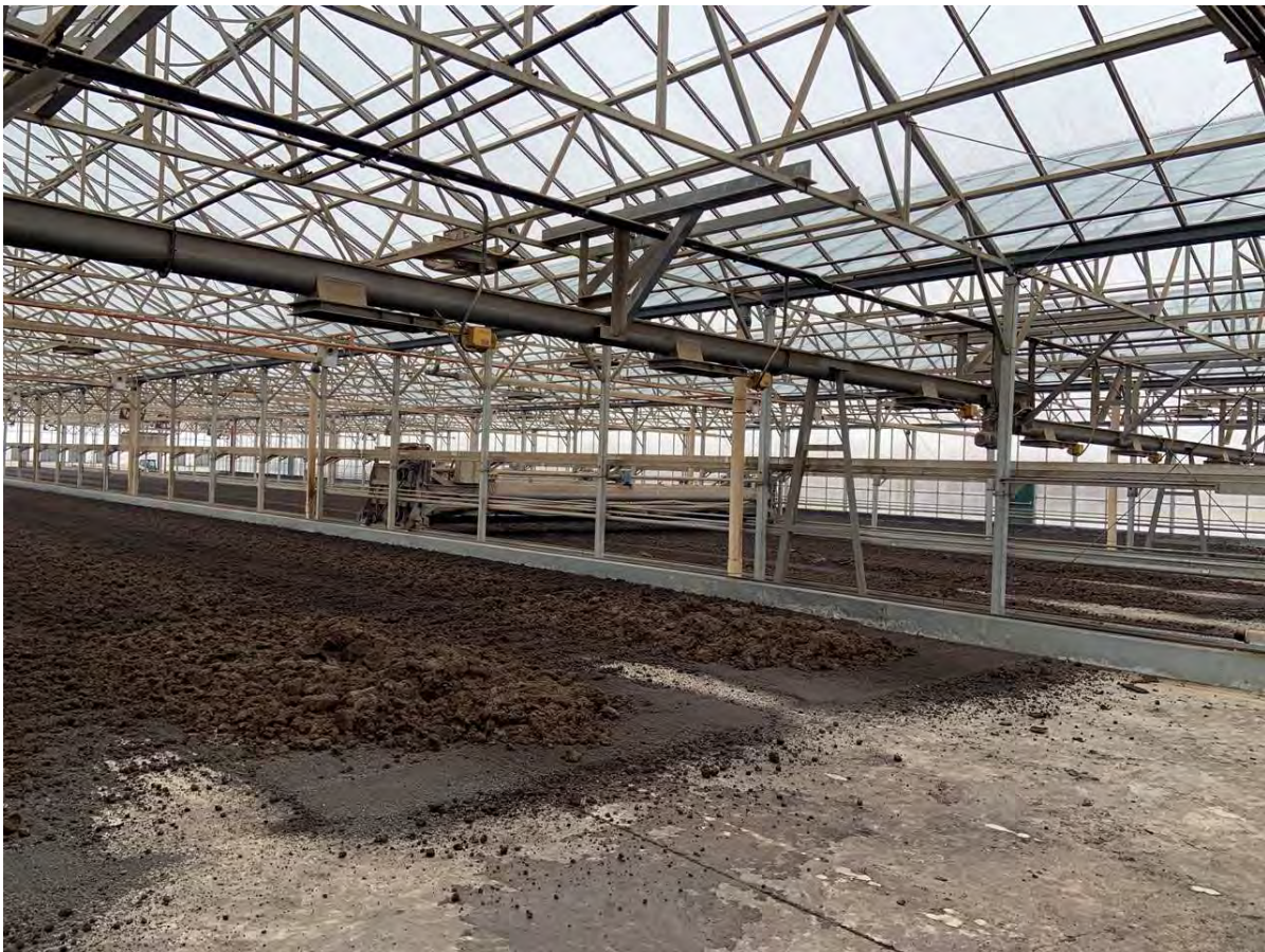
Figure 3-22: Solar Dryer Greenhouse
