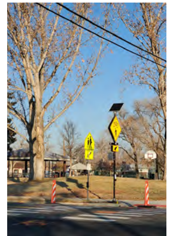
High-visibility crossing with flashing beacon
