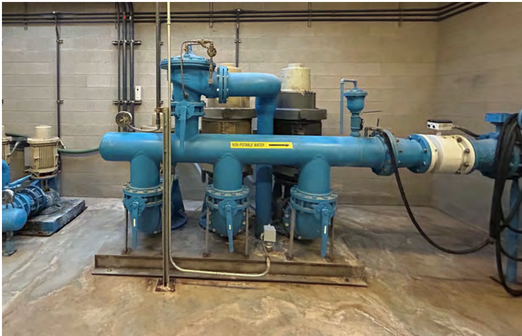
Figure 3-18: Reuse Pumping System
