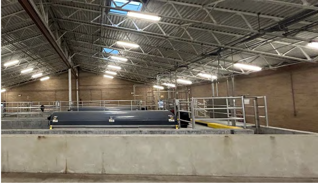
Figure 3-15: Tertiary Filters
