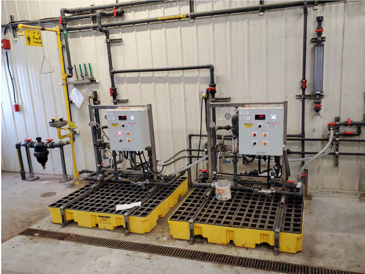
Figure 3-21: New Polymer Injection System
