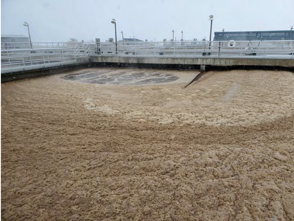
Figure 3-6: Oxidation Ditch Foaming – High MLSS
