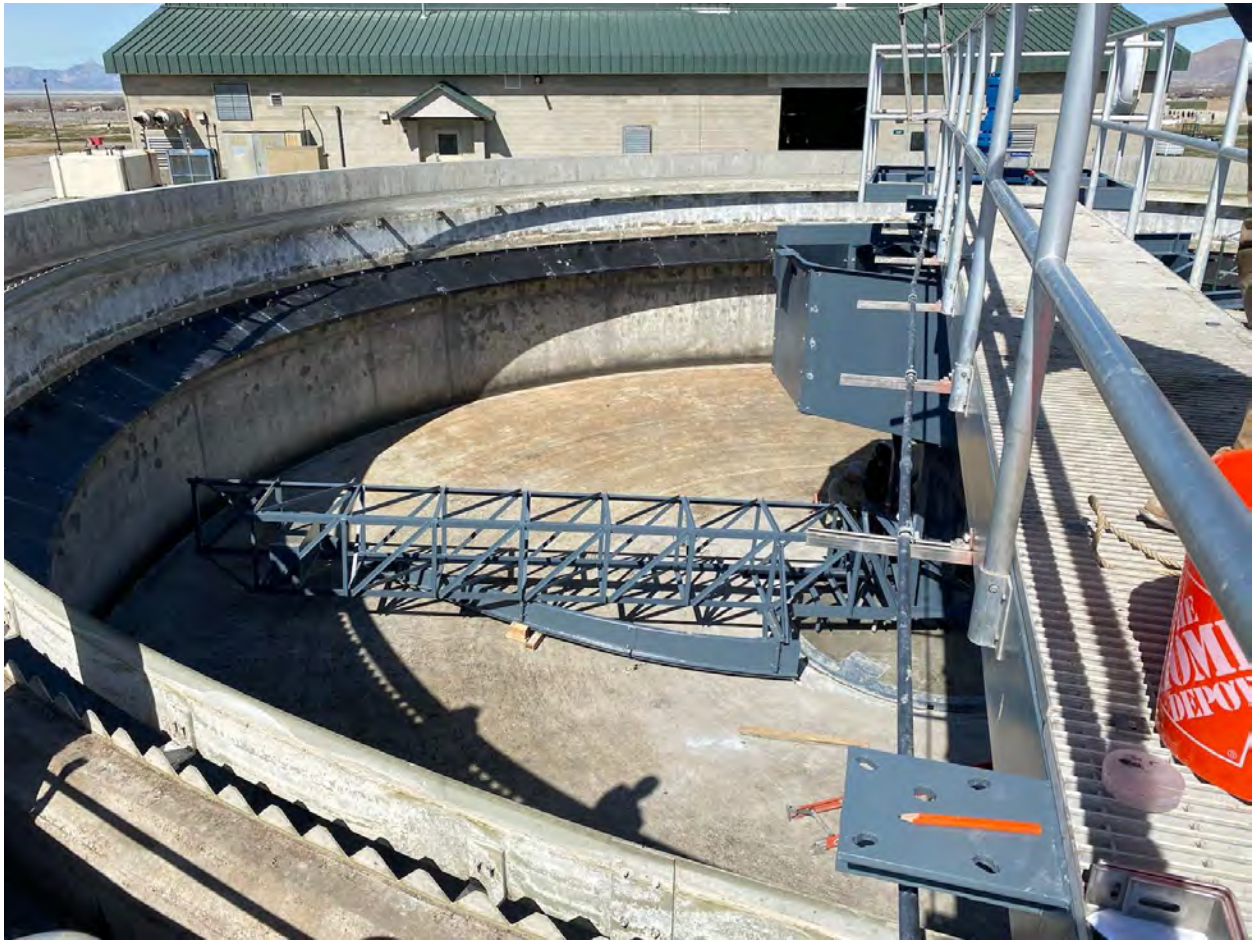
Figure 3-11: New Internal Mechanism in Clarifier #1
